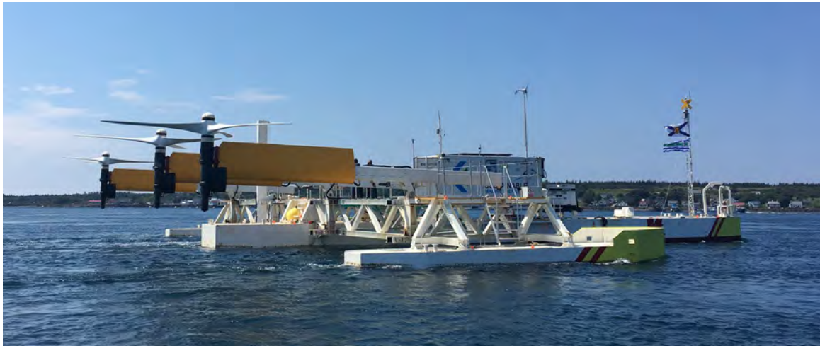
Figure 3. SME's PLAT-I platform installed in Grand Passage, NS
